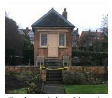
Over the years the base of the wooden balustrade has rotted away and become unsafe. Thanks to a NHLF grant, it has been repaired to its original state, but with extra protection from water at the base of the timbers.
